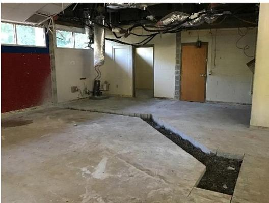
Saw Cutting for New Water Lines
